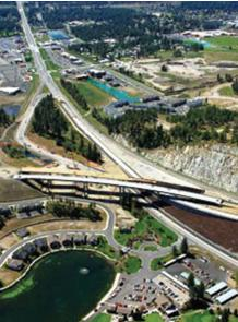
US 395 North Spokane Corridor – Spokane, WA Corrosion-resistant 1.5" diameter by 18" pavement dowel bars using ChromX® steel. Constructed 2011
