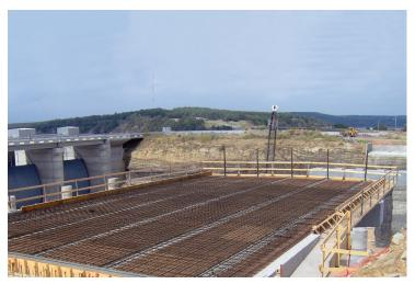
State Hwy 100 over Illinois River Lake Tenkiller Spillway - Vian, OK Bridge - ChromX® products were used for abutments, columns and deck (75 ksi design except precast elements). Constructed 2006
