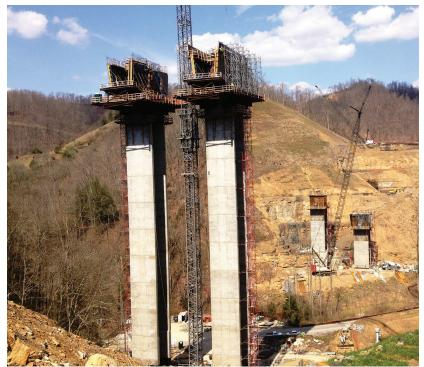
Route 460 Connector, Coal Fields Expressway Bristol Co., VA ChromX® products used for pier table (75 ksi design) and bridge deck. Tallest bridge in Virginia. Completed 2013
