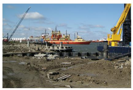
Northern Expansion at Port Fourchon, Grand Isle, LA Oil field service docks - drill shaft piles and caps utilized ChromX® (100 ksi design). Constructed 2009
