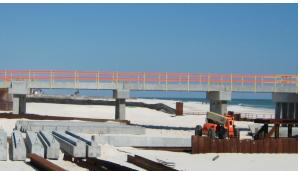
**Gulf State Park Fishing Pier - Gulf Shores, AL** 1,540 ft long precast piling and substructure built with ChromX®. Constructed 2008
