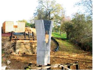
**Light Rail Bridge over Alder Creek - Folsom, CA**Bridge - ChromX® used in abutments, columns and girder (100 ksi design).
