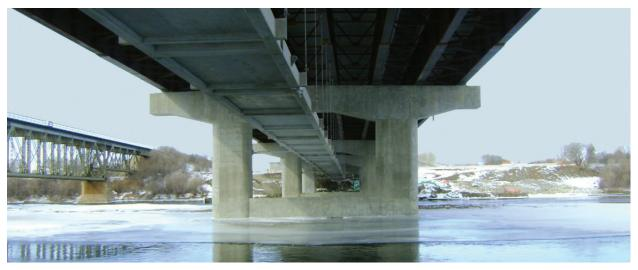
Circle Drive over South Saskatchewan River - Saskatoon, SK, CAN  ${\sf Chrom}X^{\tt @}$  steel used to construct six-lane bridge deck and columns. Constructed 2012
