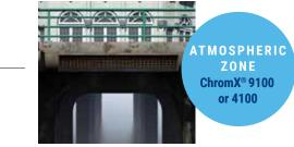
A marine atmosphere is very corrosive due to chloride exposure from salt spray, salt fog and salt mist. For atmospheric pier members in marine environments designers should consider using ChromX 4100 or 9100 depending on the target service life for the structure.
