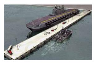
REFERENCE: New Technology Proven in Precast Concrete Modular Floating Pier for U.S. Navy, PCI Journal (October 2005)
