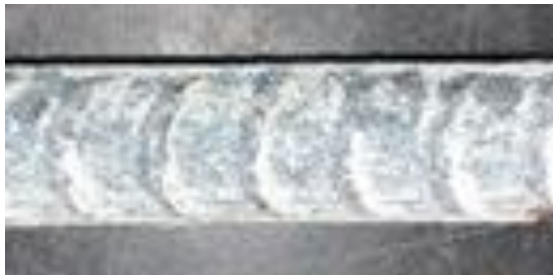
Figure 3.85: Conventional reinforcement from Cow Creek deck panel. Core taken in uncracked concrete.
