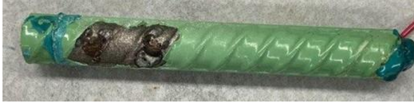
Figure 3.17: Rapid Macrocell Test. Specimen ECR2-UV-200-3 anode bar after disbondment test
