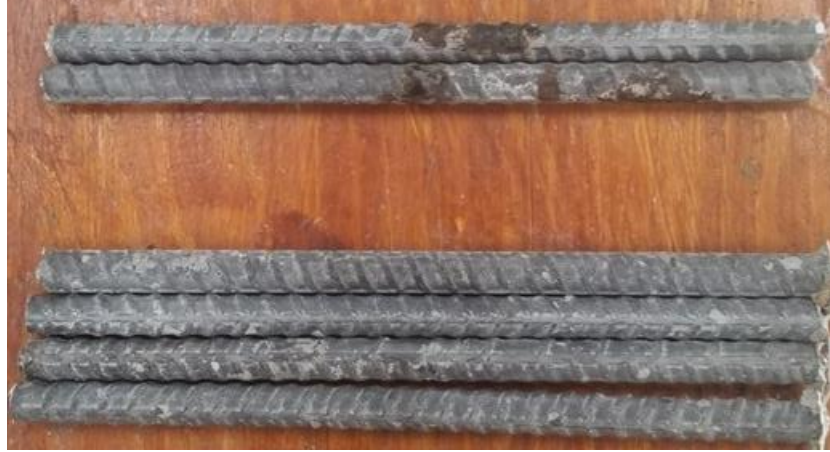
Figure 3.66: Southern Exposure test. Specimen A1035-Xypex-1 after 96 weeks of testing. Top mat (top) and bottom mat (bottom).
