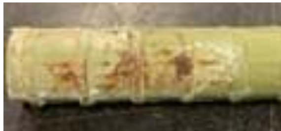
Figure 3.86: ECR from Cow Creek deck panel. Core taken at a crack location.
