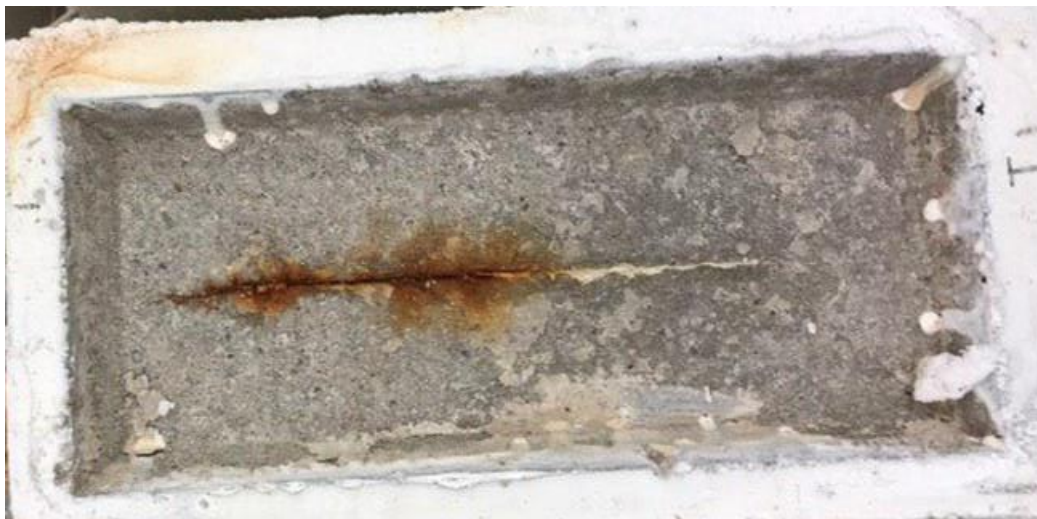
Figure 3.43: Cracked beam test. Surface staining on specimen with conventional reinforcement.
